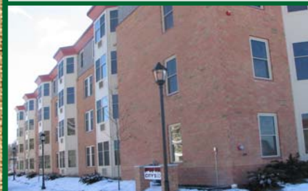
City's Edge Condominiums, South Burlington
